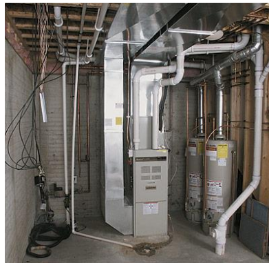
Rough-in for Mechanical Systems
