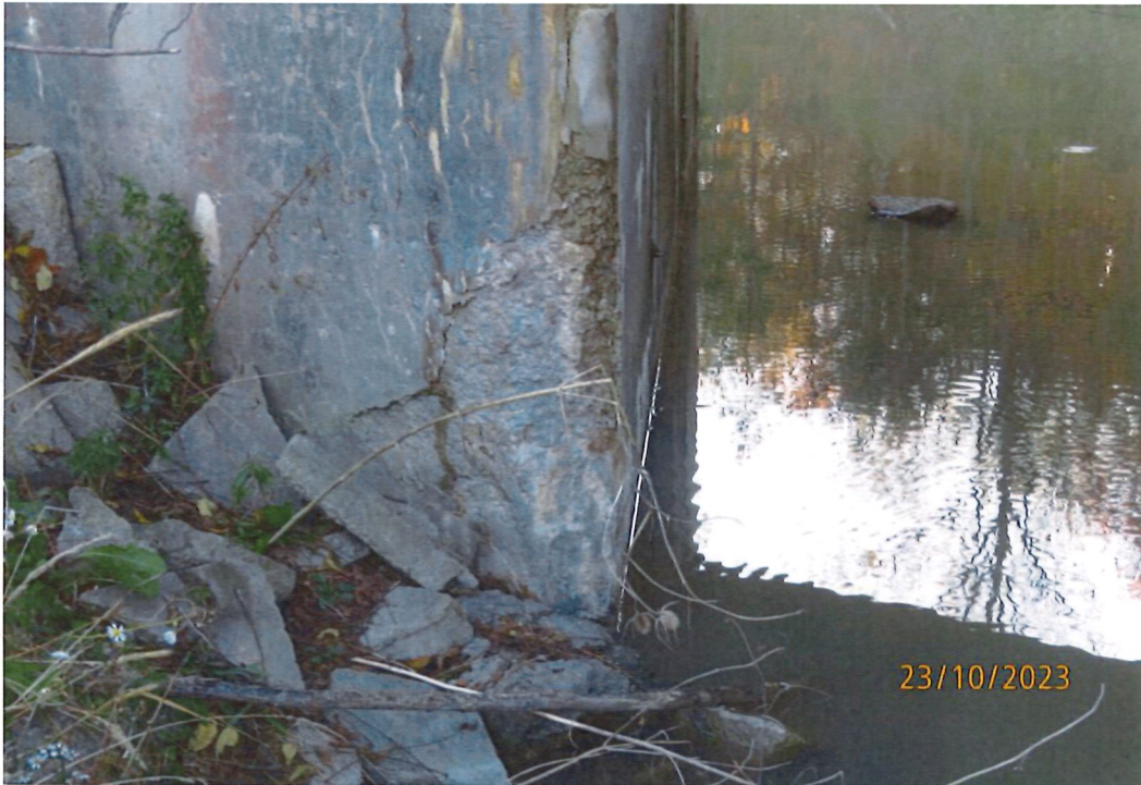
Concrete Deterioration on North Abutment Base
