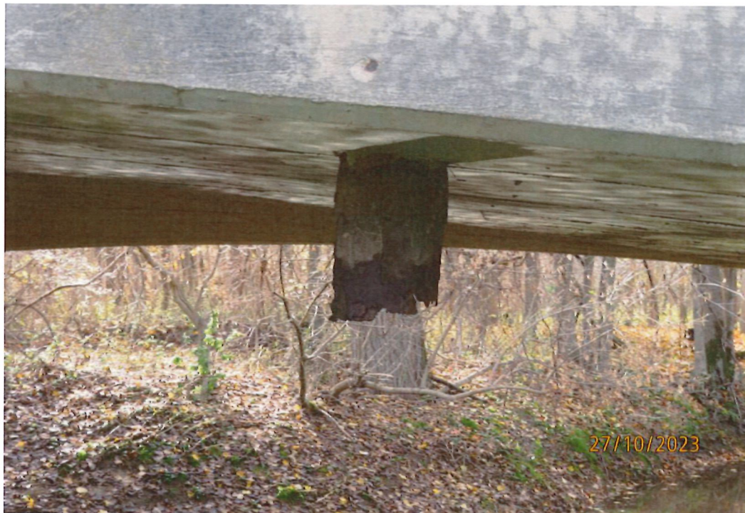
View of Deck Drains
