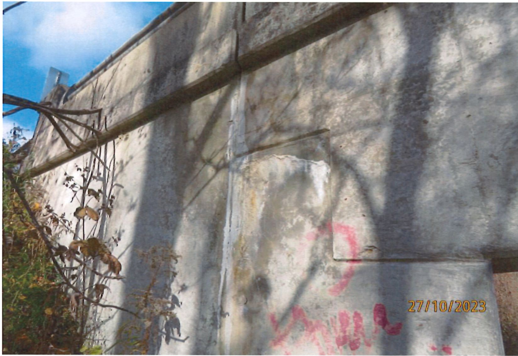
Efflorescence on Northwest Corner
