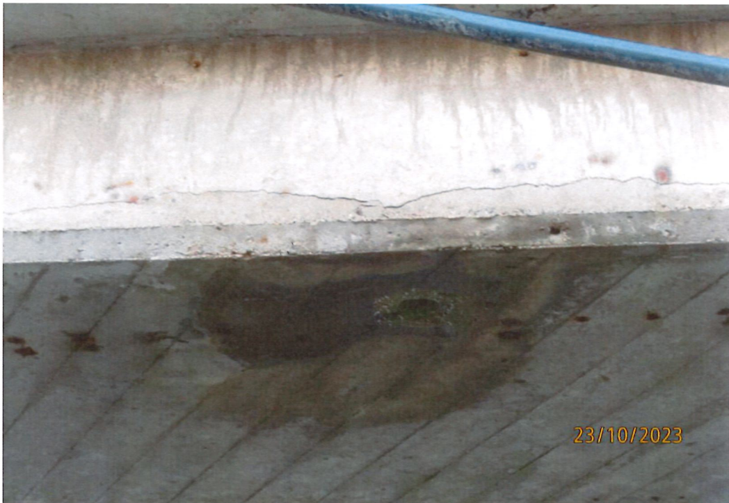
Concrete Deterioration on North Soffit
