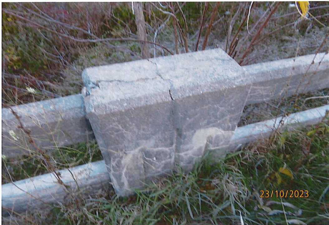
Concrete Deterioration on South Side
