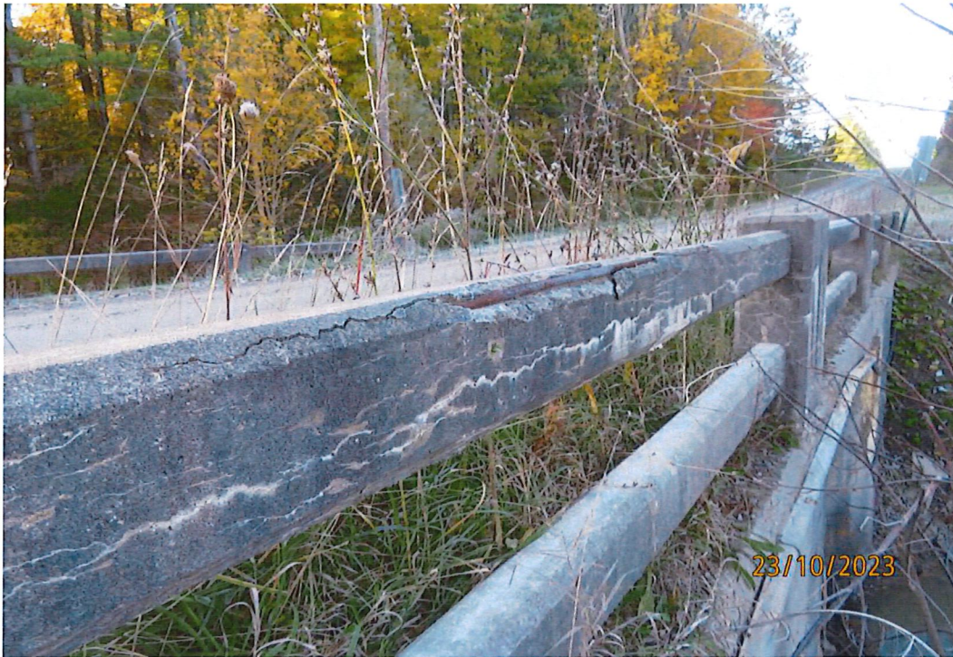
Deterioration on Railings on North Side
