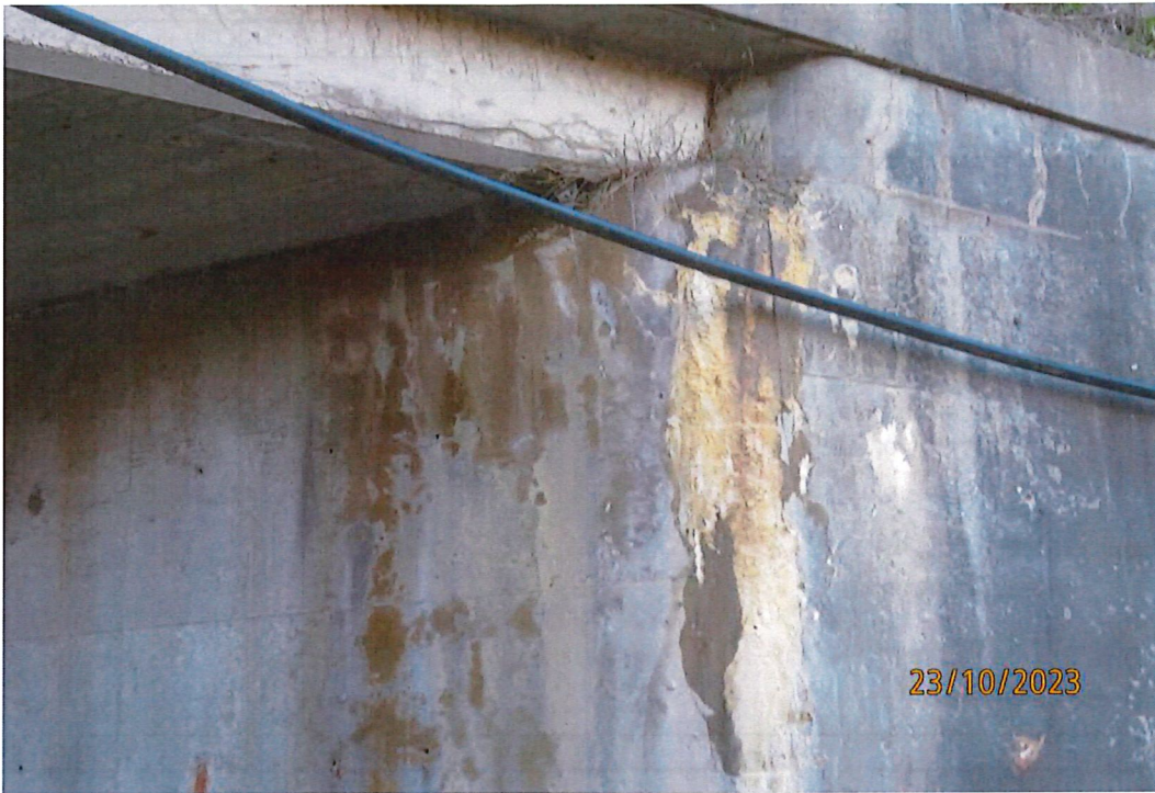
Efflorescence on North Side
