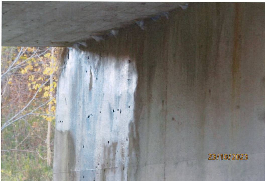
View of Concrete Deterioration on Underside of Bridge
