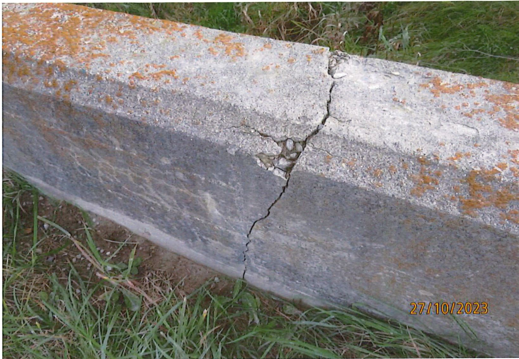
Minor Cracking and Deterioration on South Headwall
