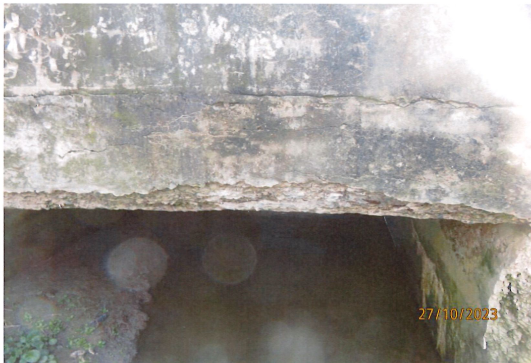
Concrete Deterioration on Outlet Side - Alternate View
