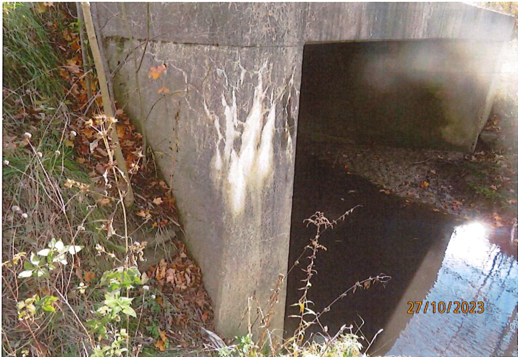
Efflorescence on Southwest Corner
