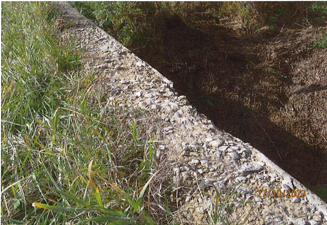
Concrete Deterioration on Top of Headwall
