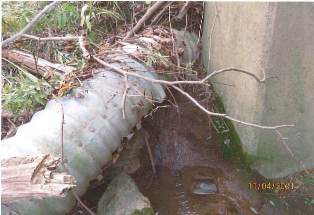
View of Rusting Outlet Pipe in Southwest Corner - File Photo
