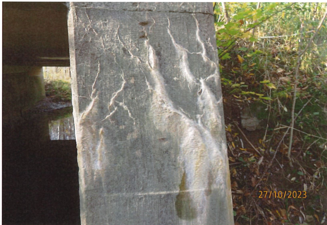
Efflorescence on Northeast Corner
