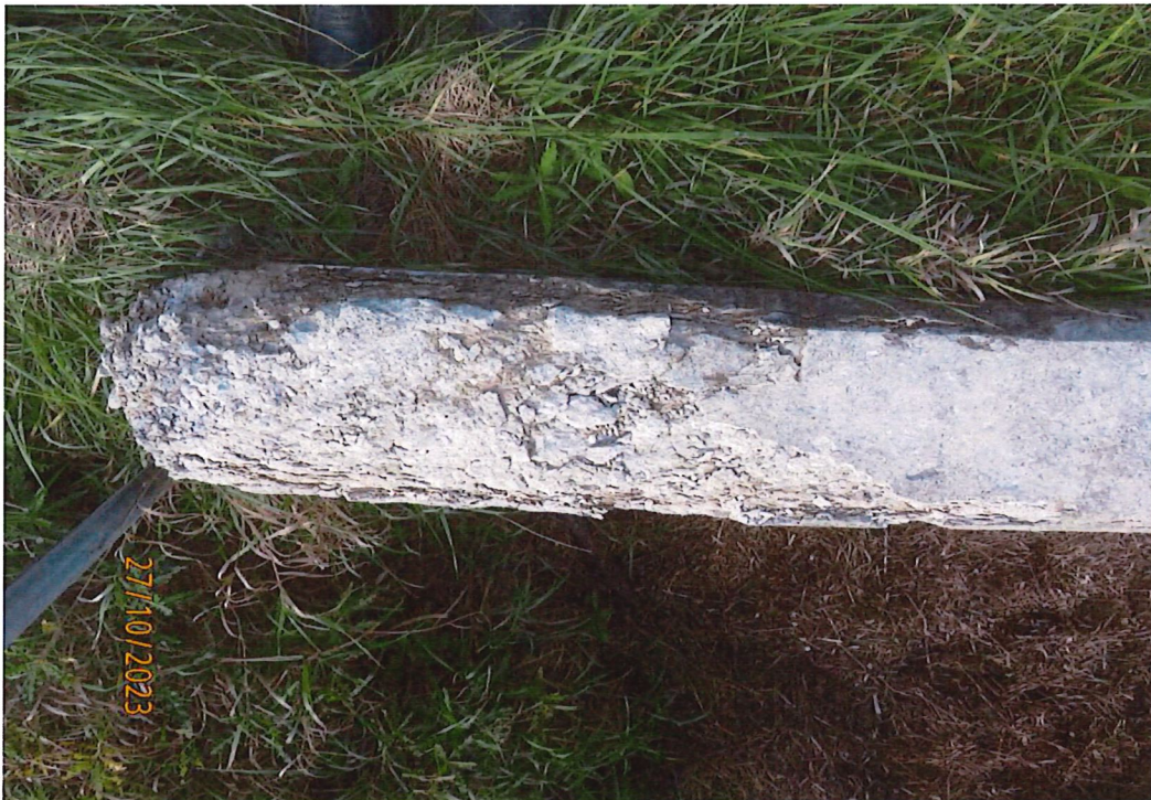
Concrete Deterioration on Southwest Corner
