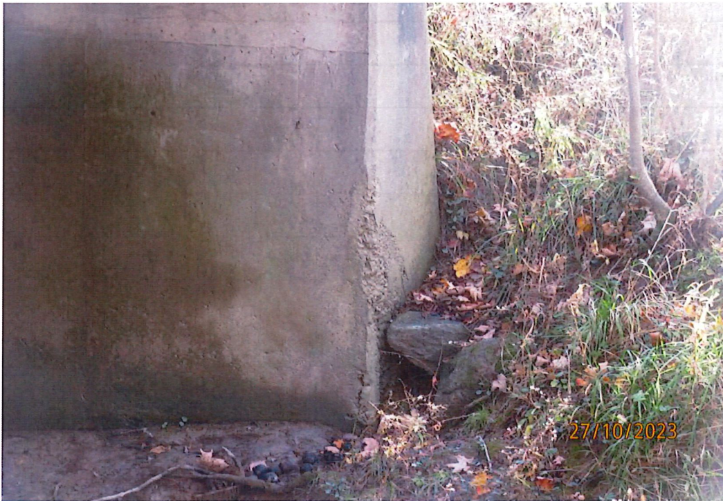
Concrete Deterioration on Southeast Corner
