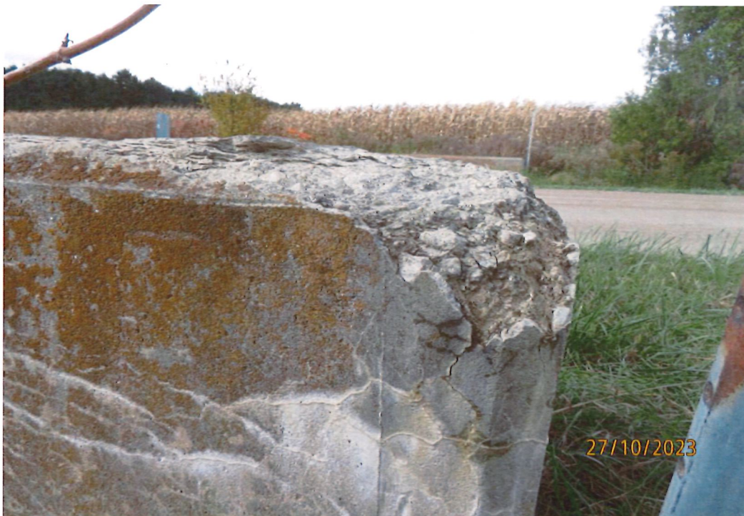
Concrete Deterioration - Alternate View
