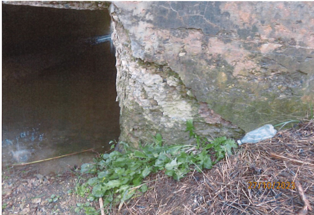
Concrete Deterioration on Outlet Side
