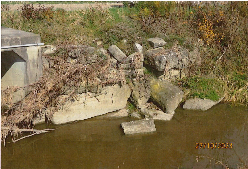
Wingwall Requiring Repair - Altenate View
